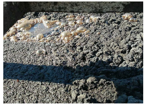
Mat of solids formed on the surface of DAF after installation of Moleaer XTB Nanobubble Generator
