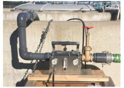
Moleaer 200 XTB installed on the outer ditch of the Village of Warrens (WI) treatment plant.
